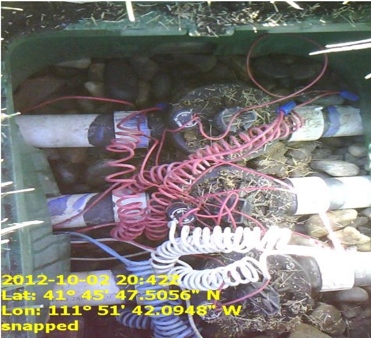
Leaking Control Valve
